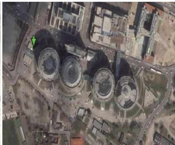
Multifunctional renovation- Vienna gasometers
